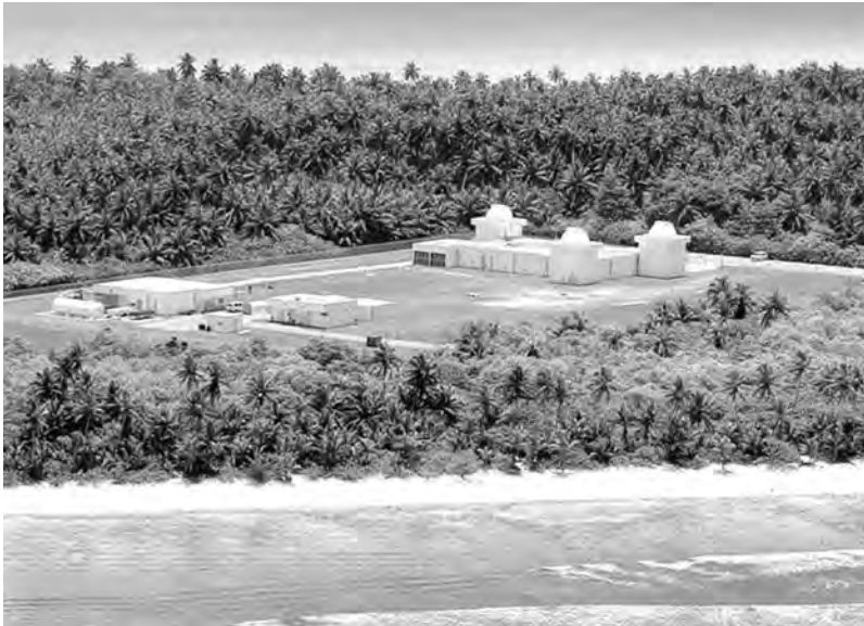
(Above) Diego Garcia GEODSS site in the Indian Ocean, ca. 1990.
